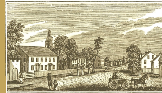
A Central View of Woodstown
